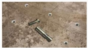
**Step 2: Move Columns Over Drop-in Anchors**
